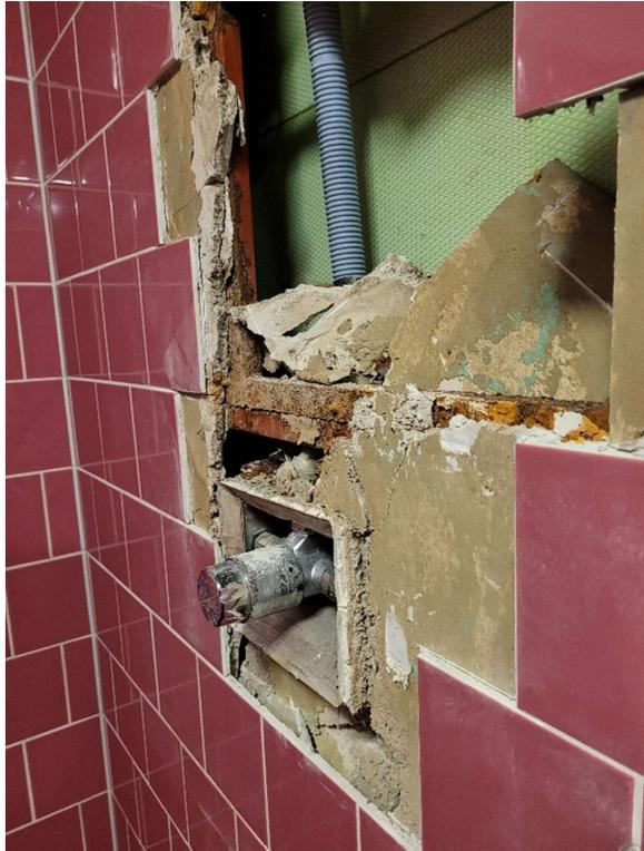
6 DU05 Vorwand Korrosion, flächig nass
